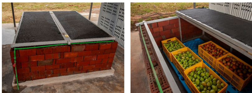
Fig. 12: The 3 rd generation Improved ZEBC at the Cold Storage Technologies Demonstration Hub
