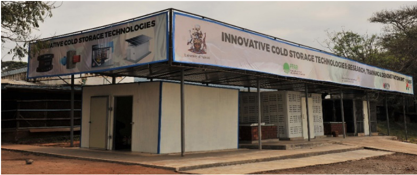
Fig. 17: The cold storage technologies hub at Upper Kabete Campus – used for research, training and demonstration
